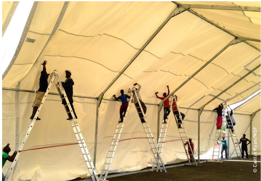
Monrovia, Liberia. Construction teams building what would become ELWA 3, the world’s largest Ebola management centre with 250 beds.
